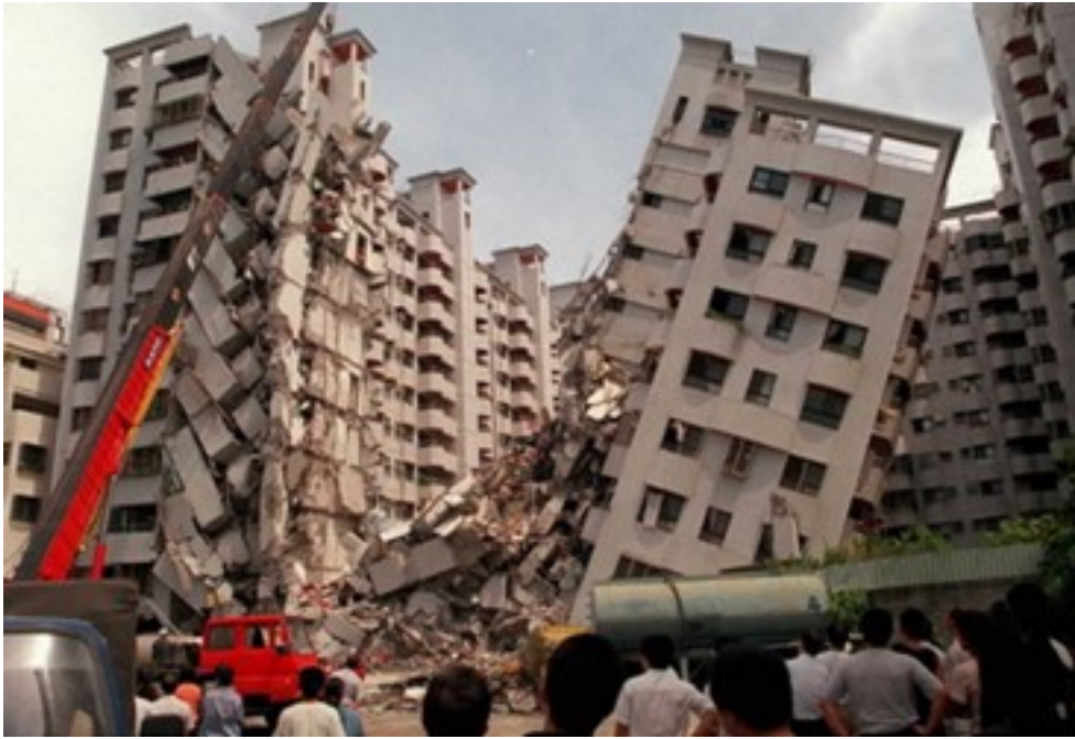
Actual building damage pattern (Pixnet, 2010)
