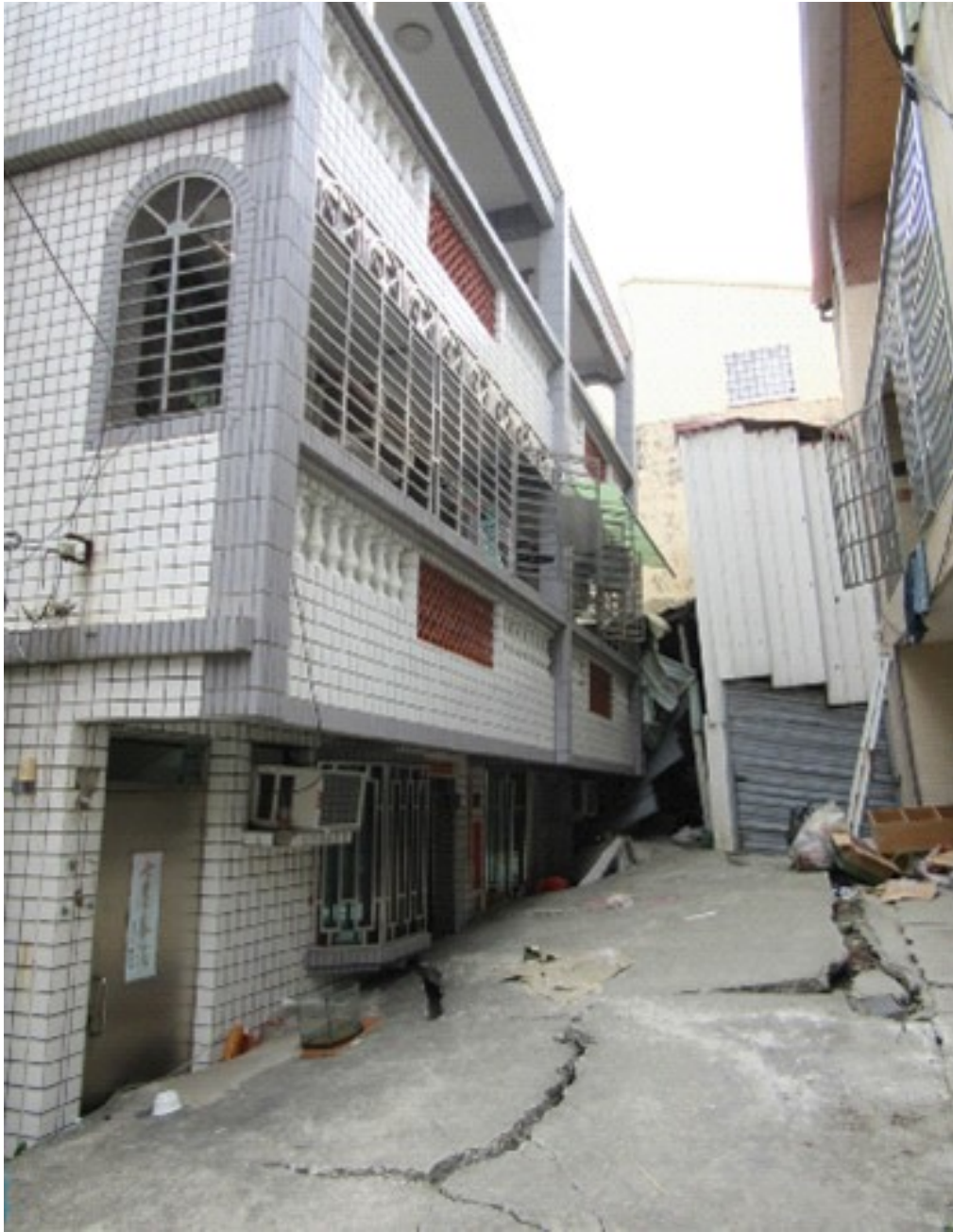
The case of misidentifying the punching shear failure of foundation as soil liquefaction (Lee, Der-Ho, 2016)
