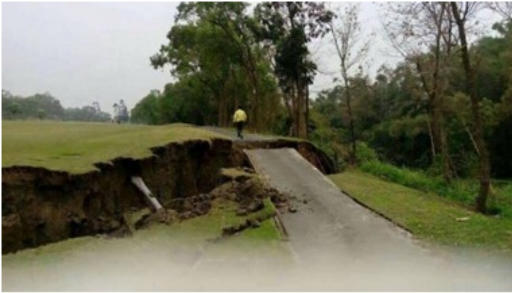
Figure 7. Striped soil liquefaction took place during Meinong Earthquake (Liberty Time Net, 2016)
