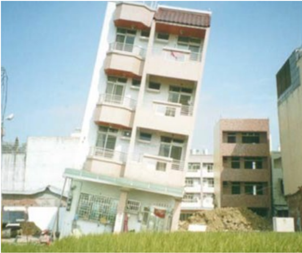
The case of misidentifying the local shear failure of foundation as soil liquefaction (Moh et al., 2000)
