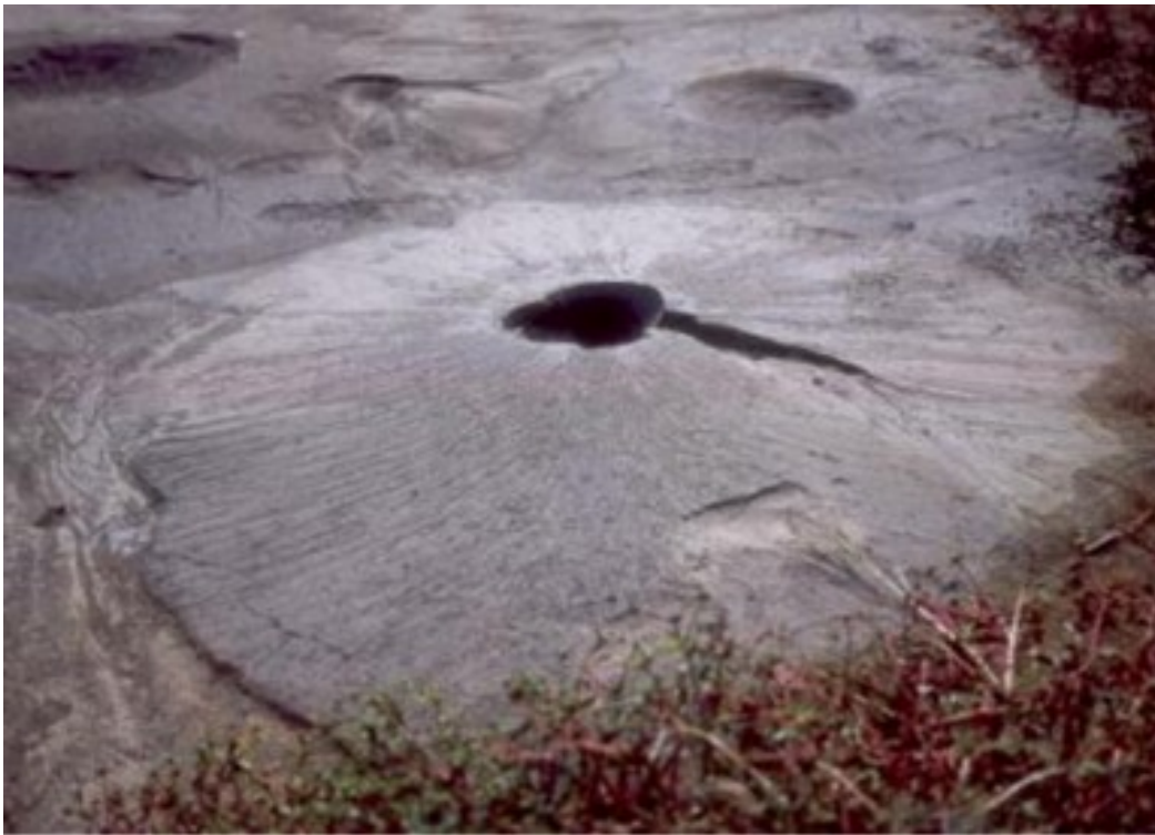
Figure 6. Tubular soil liquefaction took place during Chi Chi Earthquake (EOU Education Market, 2014)
